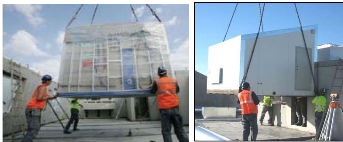
Fig. 3. Prefabricated bathroom and ventilation room modules lifted into a building site.
