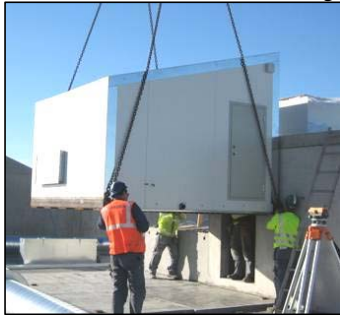
Fig.5a and Fig.5b. show the installation of prefabricated components with the crane's help.
