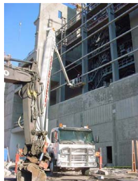
Fig. 1a. Hatch access provided through large windows Fig. 1b. Mechanized lift through wall hatches
