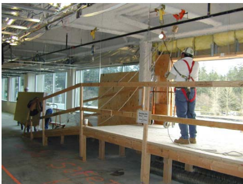
Fig. 1a. Hatch access provided through large windows Fig. 1b. Mechanized lift through wall hatches
