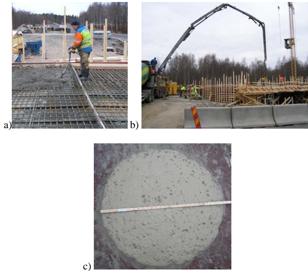
Figure 4: a) Worker using a vibrator for compacting normal concrete. b) SCC being pumped into formwork. c) Slumpflow test on SCC measuring approximately 740mm.
