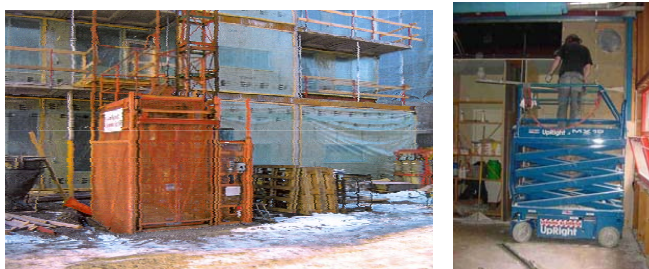
Fig. 6. Personnel and material hoist, and a scissor lift
