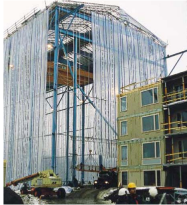
Fig. 8. A weather independent production hall with safe lifting with a traverse.
