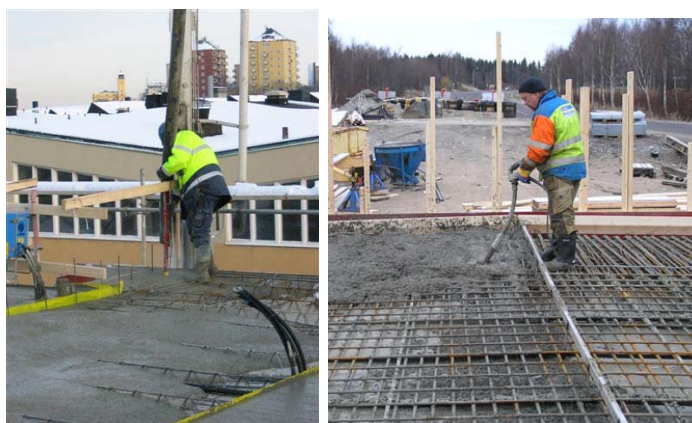
Fig. 7. Self-Compacting Concrete Casting (photo on the left) with no need to use a compacting vibrator (as seen in photo on the right).
