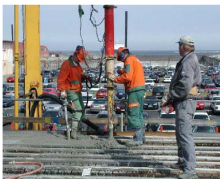
Fig. 5. Concrete cast with a remote-controlled pump
