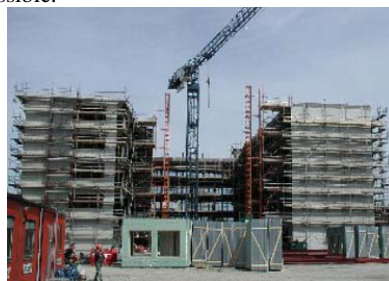
Fig.6a and fig.6b. show a ready assembled scaffolding system to provide a safe working platform and an effective placement of the crane which should be designed in site layout to minimize risks on workers.
