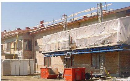
Fig.6a and fig.6b. show a ready assembled scaffolding system to provide a safe working platform and an effective placement of the crane which should be designed in site layout to minimize risks on workers.
