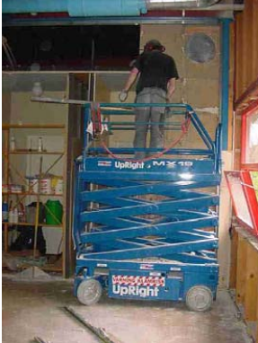
Fig.3a. Indoors work tasks done on scissor lift Fig.3b. Heavy prefab materials in indoors workspace require mechanical lifting device
