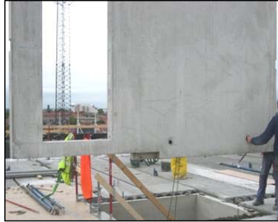
Fig.5a and Fig.5b. show the installation of prefabricated components with the crane's help.
